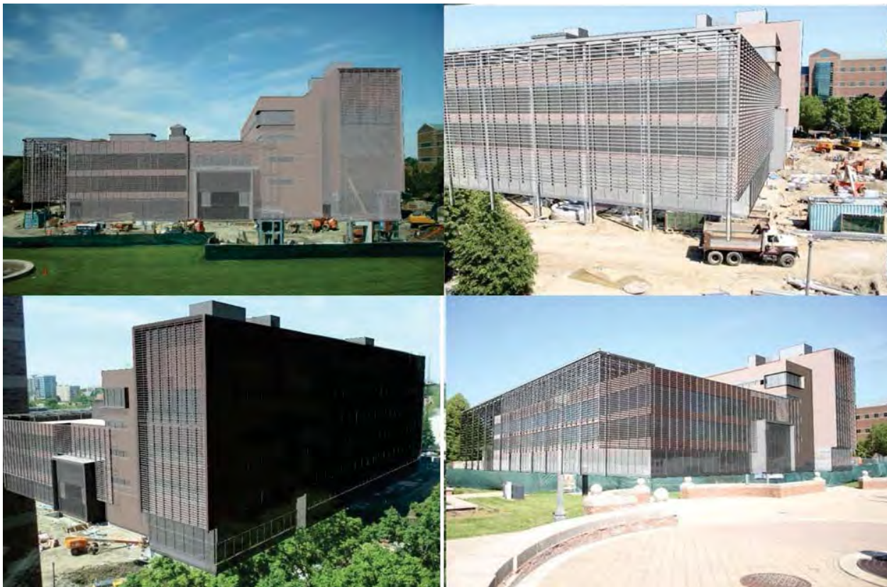
Figure 7. BIM-assisted SfM: enhanced accuracy of overlaying BIM on site images.
