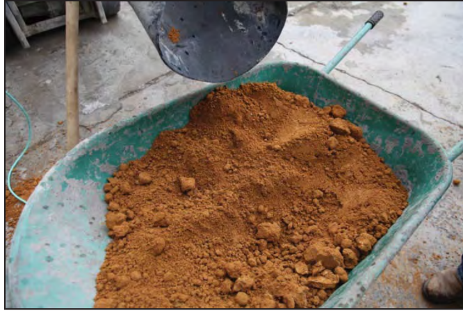
Figure 3. Louisiana clay prior to CEB production
