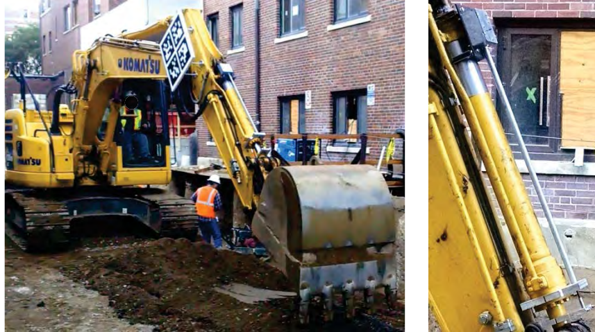
Figure 18. Cable potentiometer prototype installed on excavator
