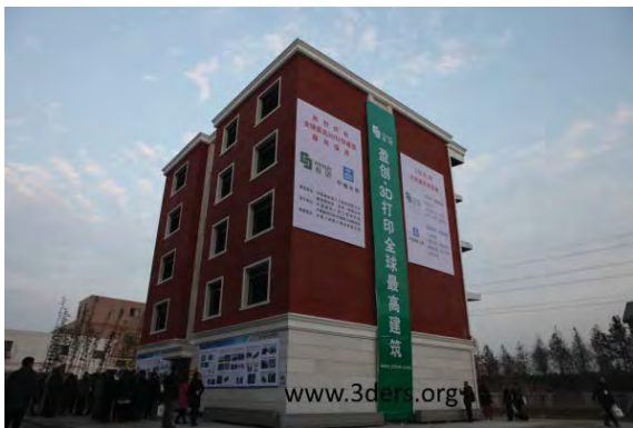
Figure 4 – A 3D printed five-story apartment block (Charron 2015)
